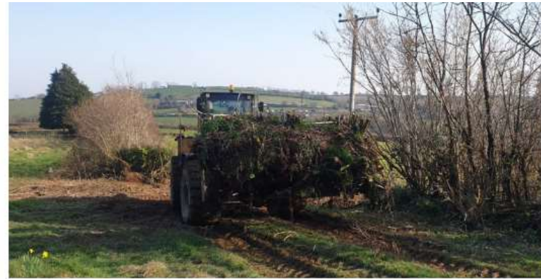
Plate 8: Large section of hedge being translocated by tined loader
