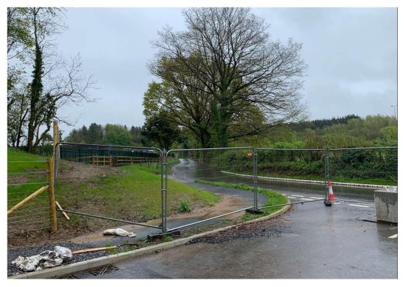
On the way back, some members of the group commented on the pleasing result of the mix used to make up the final wearing course of the road. Barry explained that the mottled effect was the result of the mix of materials, including aggregate from Glendinning's other quarry at Pigsdon.
