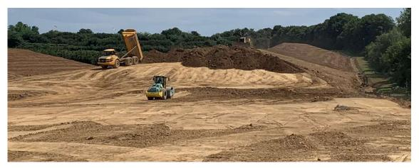
A dump truck has just dropped its load, and the dozer is starting to level the heaps of overburden. The roller is in the foreground, getting ready to compact the levelled surface. The completed section of bund is visible in the background.
