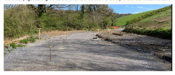
Barry explained that the alignment towards the top section of Waye Lane followed closely the winding route of the previous farm track to help keep the rural feel of the road. In addition, hedgebanks will be built and planted as close as possible on both sides of the road to complement the existing hedgebanks that were retained or relocated to accommodate the road.
