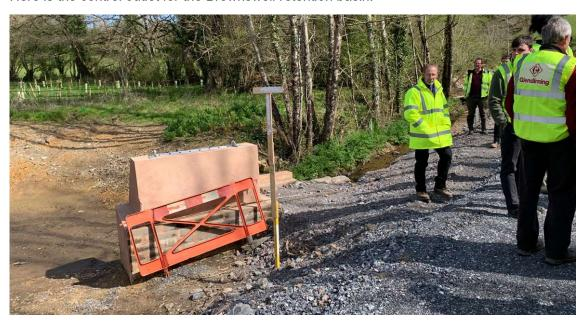
Here are some shots of the base layer surface of Waye Lane. The level of the eventual finished surface will be one metre below the tops of the wooden pegs either side of the road and the metal pegs show the proposed curb line.
