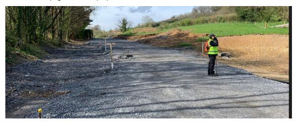
The metal pegs marking the curb line can also be seen at the top end of this middle section.
